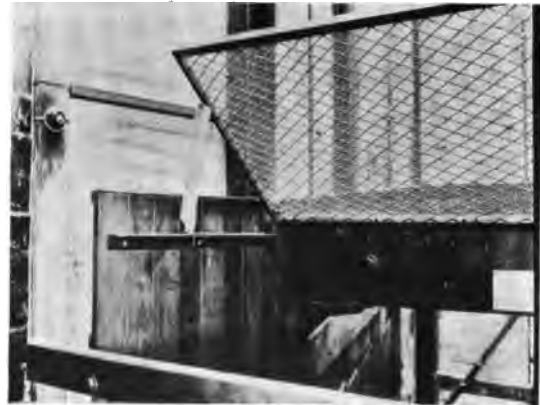
Fig. 3. Hinged Cover for Elevator Car. This will release automatically if it should catch as the car descends.
